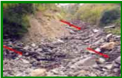
The velocity of runoff and landslide has been checked by cross sausage wall
