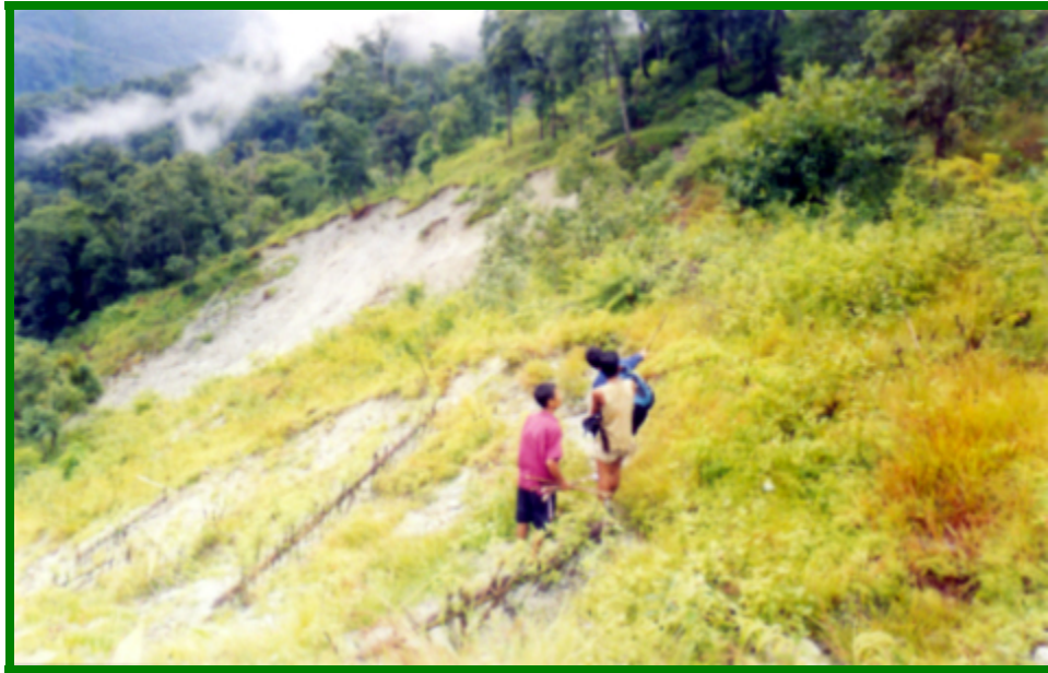
Plantation of cuttings across the slopes of landslide
