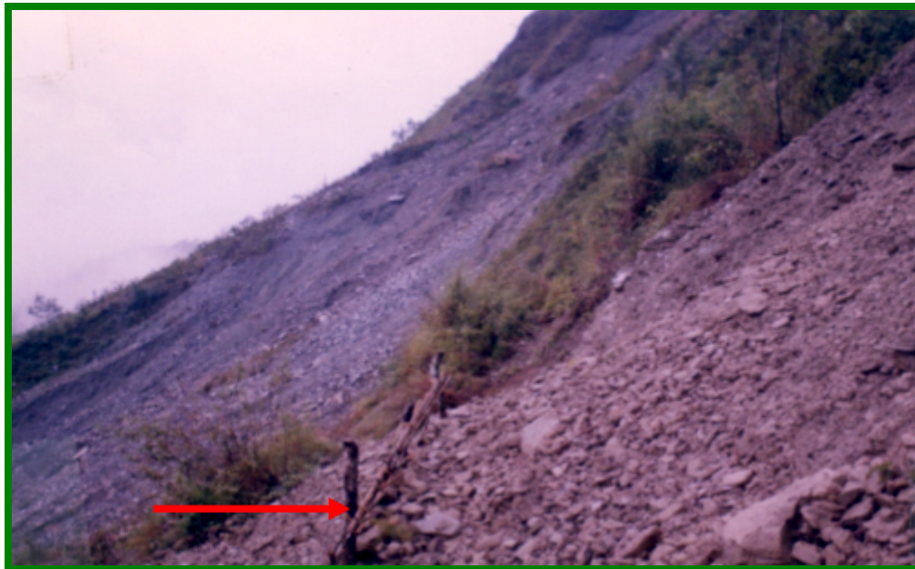
Toppled Gravelly Loamy Sand partially checked by bally benching
