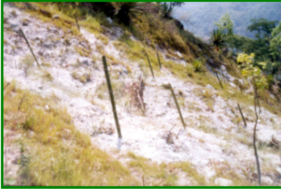
Bamboo plantation in landslide
