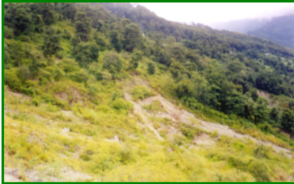
Vegetation of Donok Landslide
