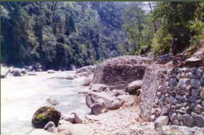
Training of Turbulent Torrent with Sausage and Spur structures
