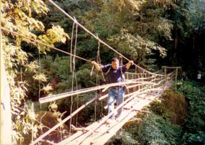
Crossing Broken cane Bridge - Life & death challenge
